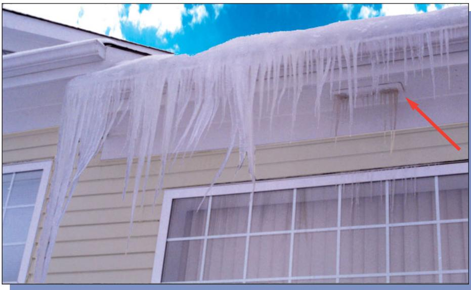
Figure 4 — An example of severe ice damming. Icicles hanging from the soffit vent (arrow) indicate melt water has penetrated the roofing and roof sheathing.
