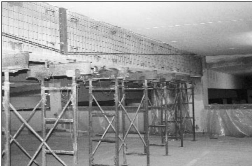
*Figure 1 - External post-tensioning repair installed with wire mesh in place prior to gunnite application.*
