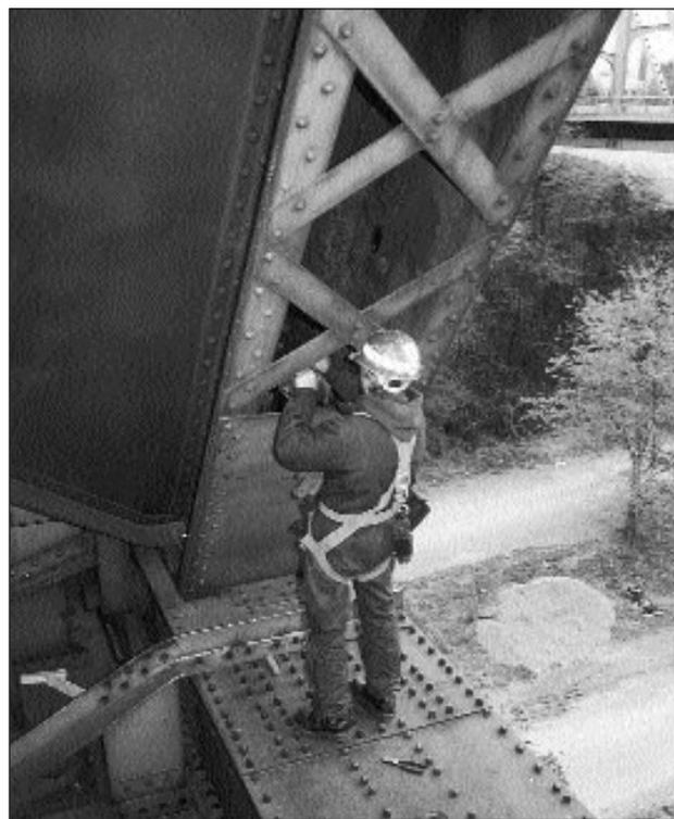
Figure 3 - Technician Installing Strain Gages.
