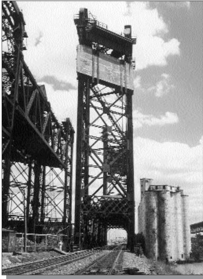
Figure B – Two adjacent lift bridges, one with span raised and one with span lowered. Note the large concrete counterweight.
