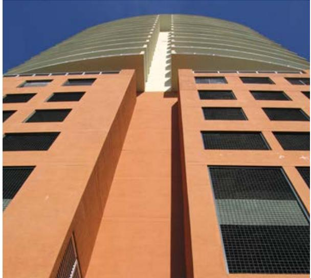
Recent RRJ investigations of stucco cladding distress on high-rise buildings in the southeast United States identified recurring problems associated with a popular method of stucco cladding installation. Engaged by building owners and contractors to diagnose the causes for the stucco cladding distress and to develop recommendations for repair of their building walls, RRJ provided professional services including:
