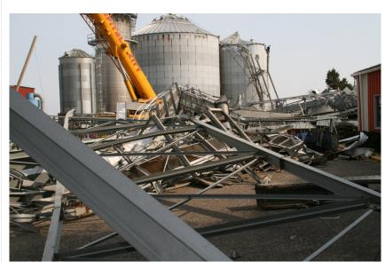
RRJ was recently retained to review the partial collapse of a grain storage facility located in the Midwestern United States. A wind storm caused the complete collapse of the elevator and conveyor system and collateral damage to the grain storage bins. Services provided included:
