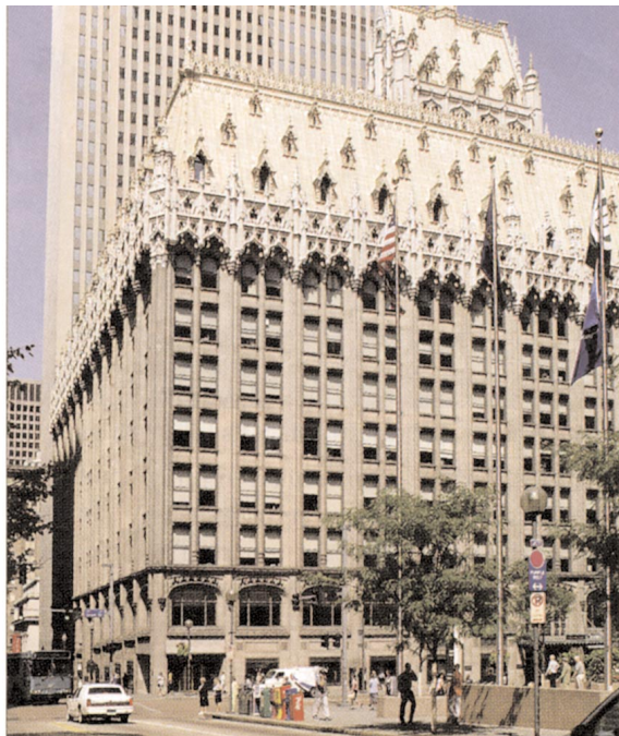
▲ Pittsburgh Gem. Leaky mansard roof repaired slowly.
