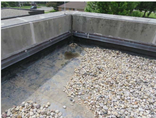
Photo 2: Past work or wind scour has moved river rock around in the more critical corner zone potentially leaving the membrane more vulnerable to uplift damage. (Raths Raths & Johnson photo)
