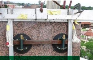
Granite panel support rig used to assist in removing, transporting, and re-installing panels
