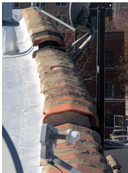
FIGURE 4. Two examples of masonry wall bowing due to lack of movement joints.
