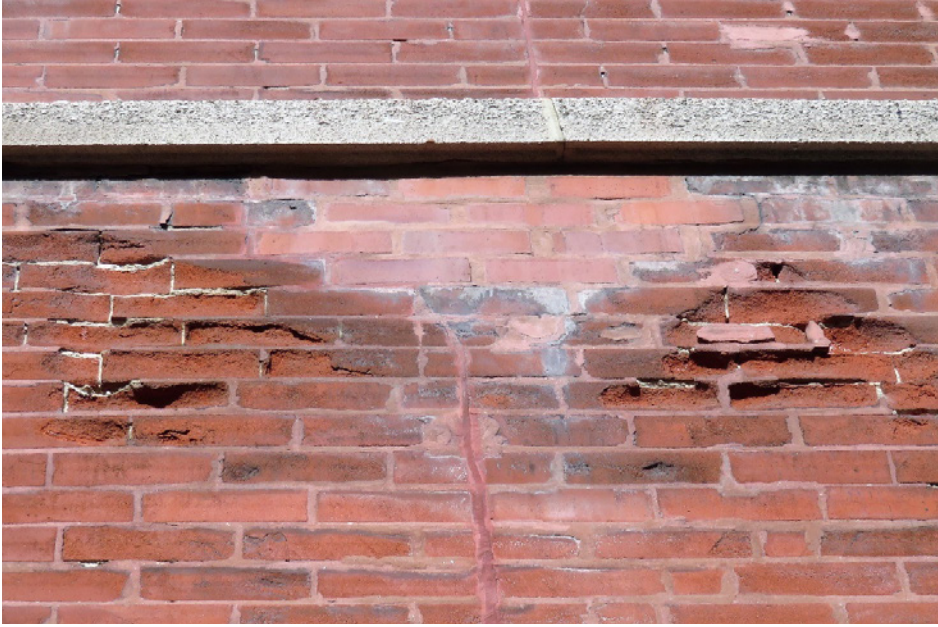
FIGURE 2. Various forms of exterior masonry wall deterioration.
