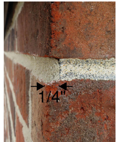
FIGURE 7. Mortar joint repointing to an insufficient depth of approximately \frac{1}{4} in. (6.4 mm).
