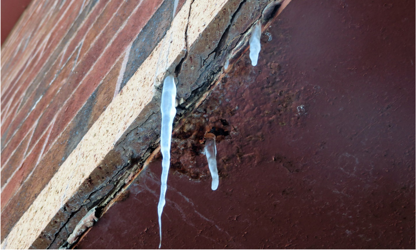
FIGURE 3. Deterioration of brick veneer from freezing and thawing cycles.
