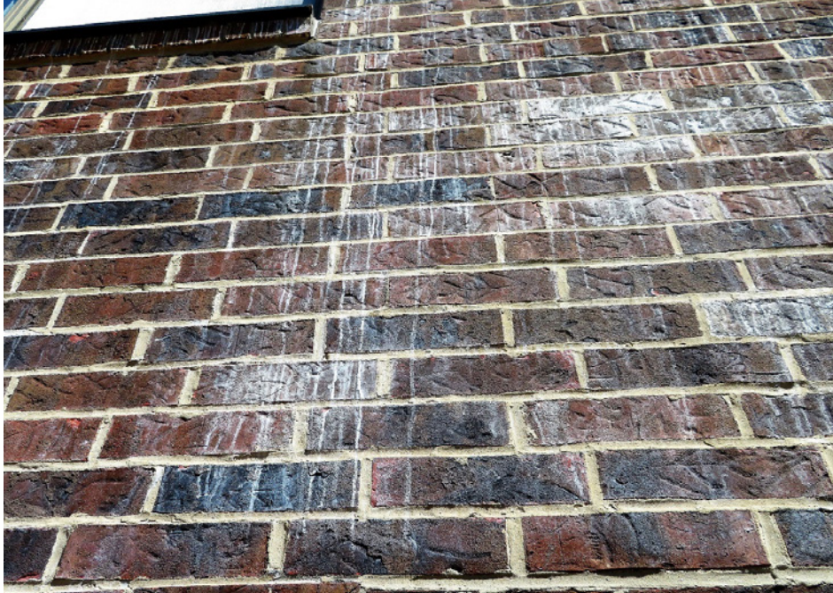
FIGURE 8. Water-repellent staining on an exterior masonry wall surface.
