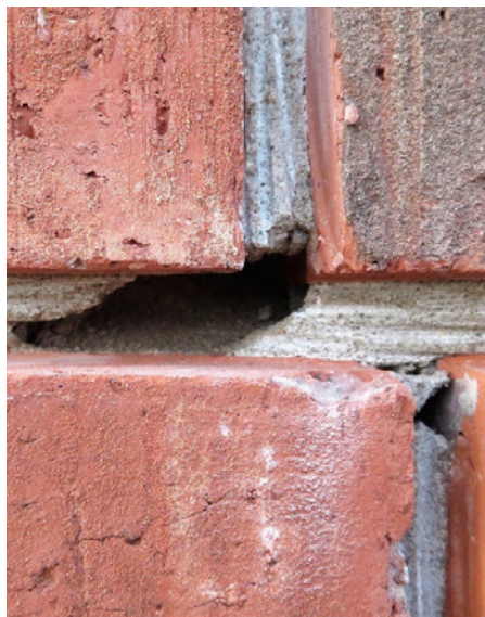
FIGURE 6. Voids in a mortar joint were uncovered following grinding during a repointing project.
