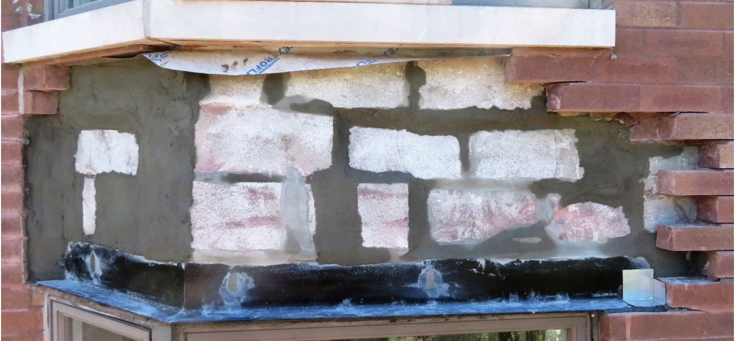
FIGURE 9. Preparation of a backup wall prior to installation of the AWB and through-wall flashing.
