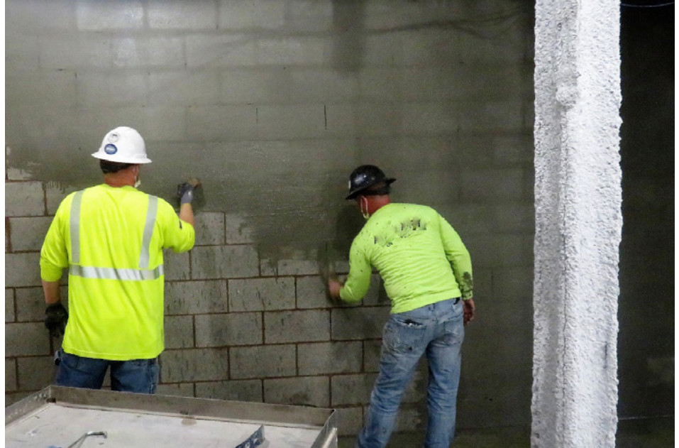
FIGURE 14. Crystalline waterproofing application on the interior side of a CMU wall.
